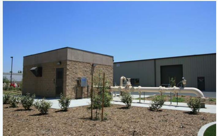
Well # 19 and the District Warehouse in the Background
