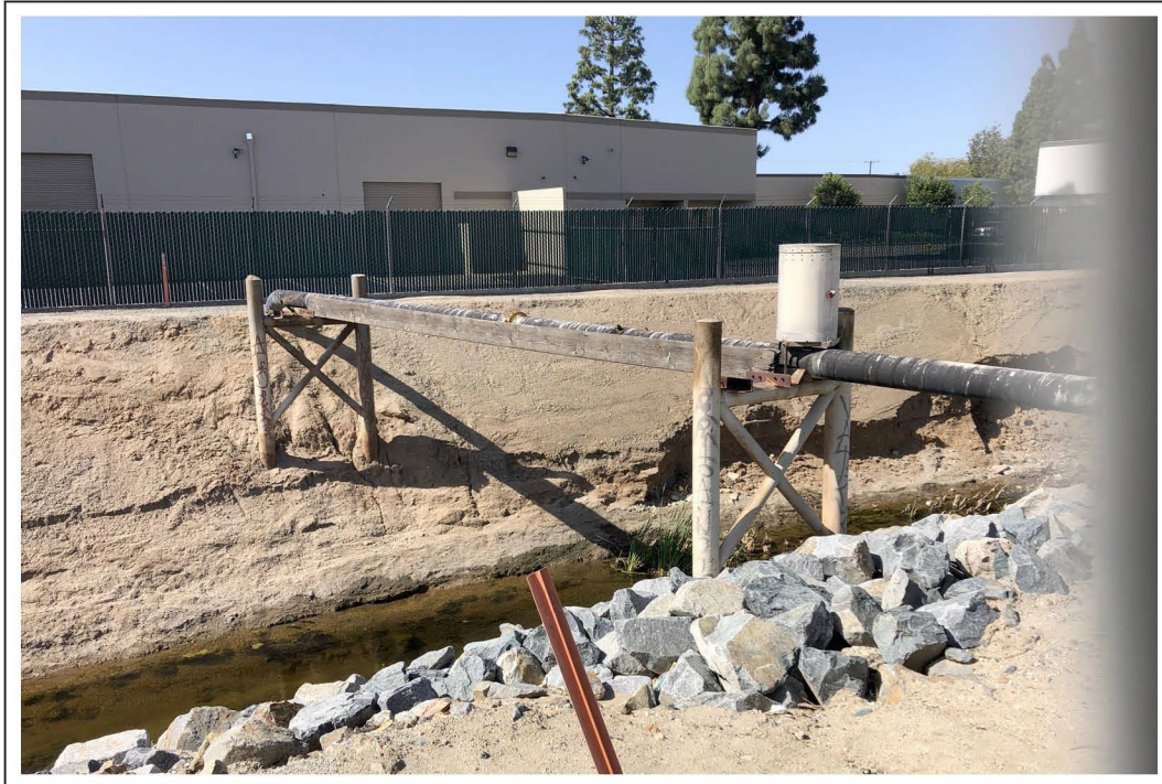
Photo 1. Existing pipeline crossing Atwood Channel. April 7, 2022.
