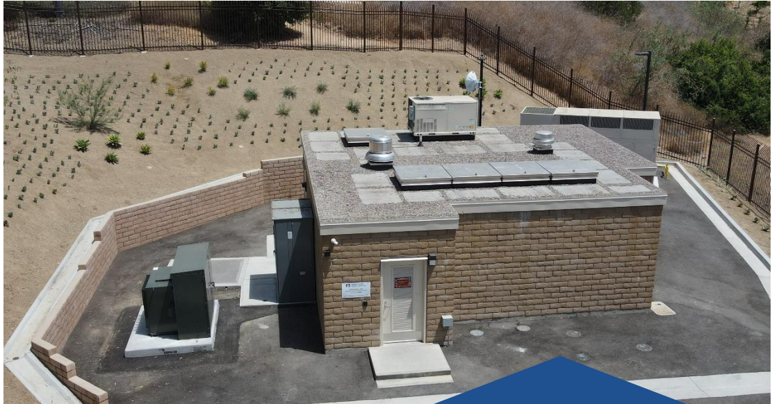
Hidden Hills B.P.S. Design Pumping Capacity: 3,600 GPM
