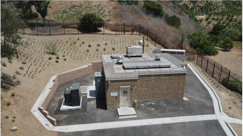
Hidden Hills Booster Pump Station
